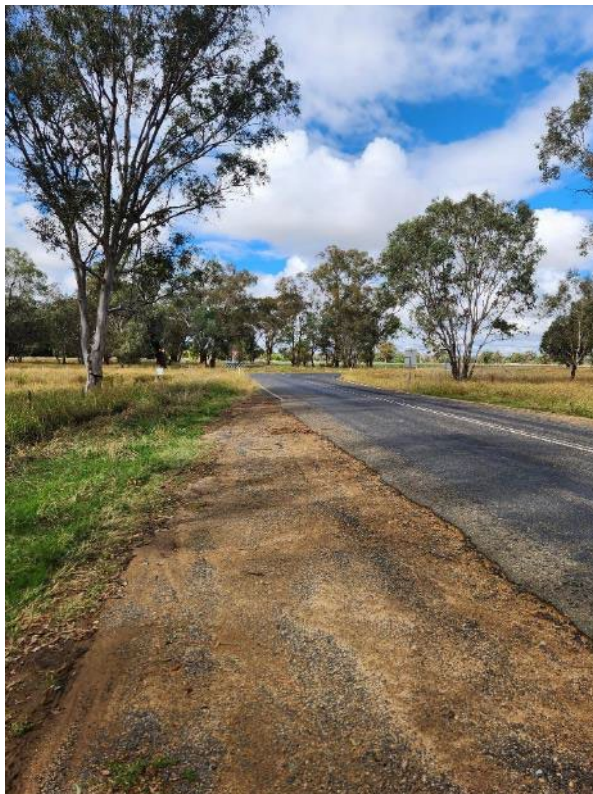
Photograph 8: Old Forbes Road Looking Towards Intersection with Henry Lawson Way from ~100 m Down Road
