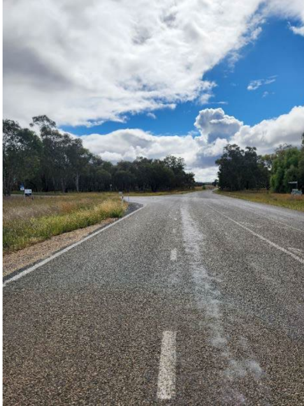
Photograph 9: Looking North Down Henry Lawson Way from the Intersection with Old Forbes Road
