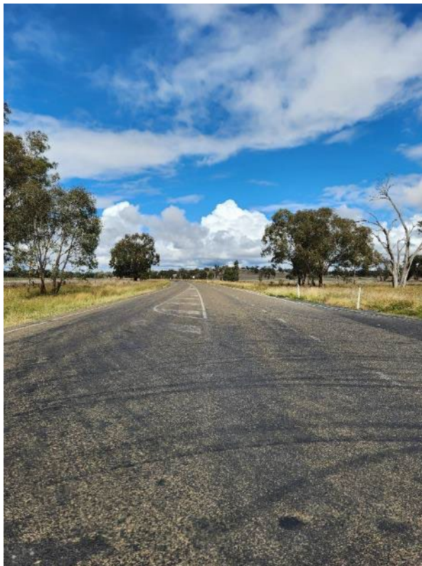
Photograph 10: Looking South Down Henry Lawson Way from the Intersection with Old Forbes Road
